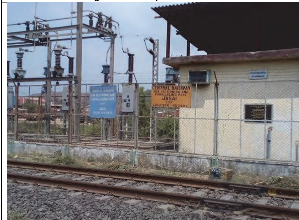
Figure 13 . Central railway line crossing the alignment of MTHL at Jasai
