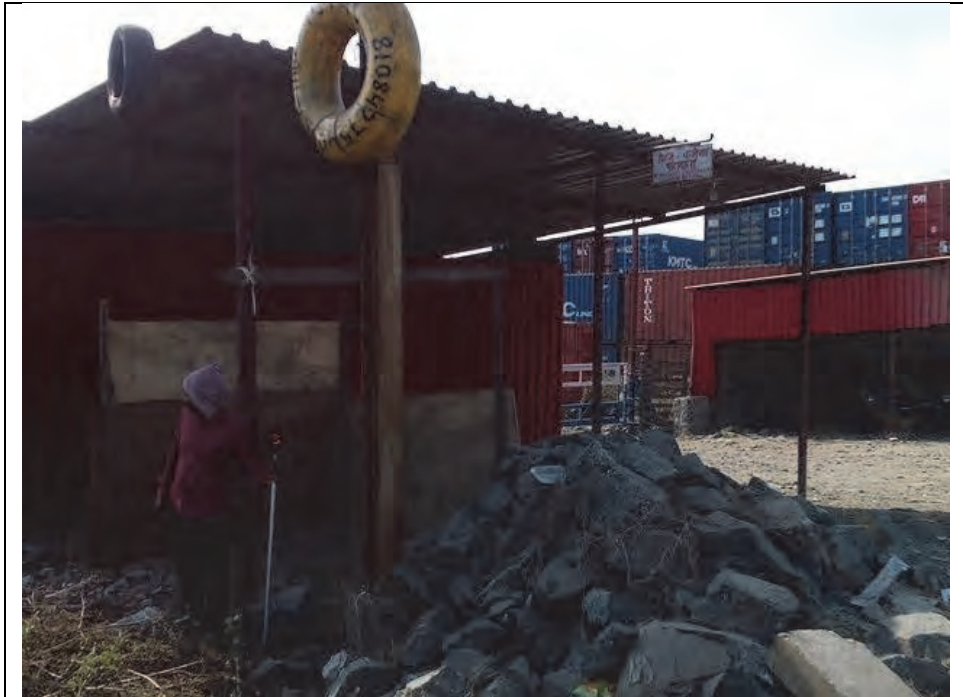
Figure 12 . Survey work at Chirle
