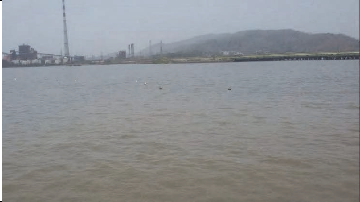
Figure 18 Pir Pau Jetty at KP5.88
