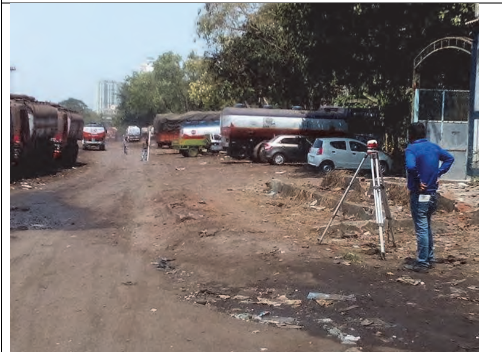
Figure 8:-topographic survey work at Seweri Site
