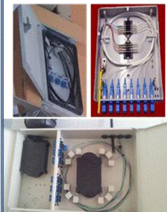
FTB for MDU located in Riser Room
